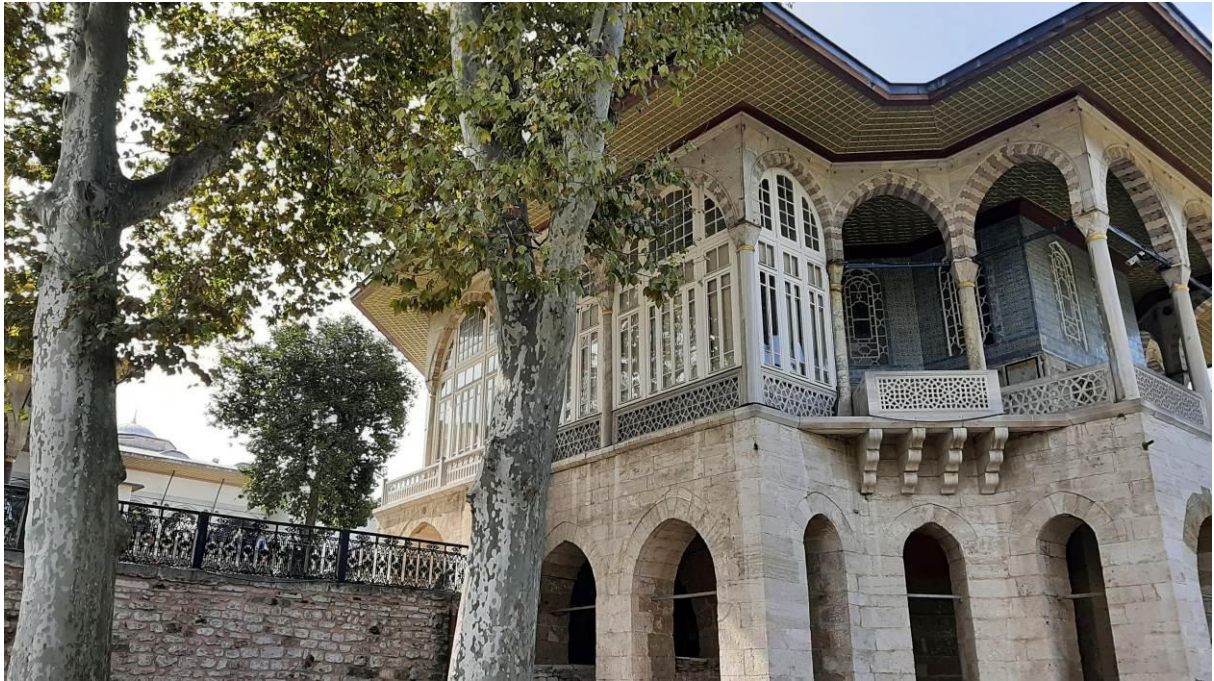
Photo 9. Topkapi Palace, dating back to 1465, is the oldest seat of government surviving in Istanbul—detail of the Baghdad Pavilion.
