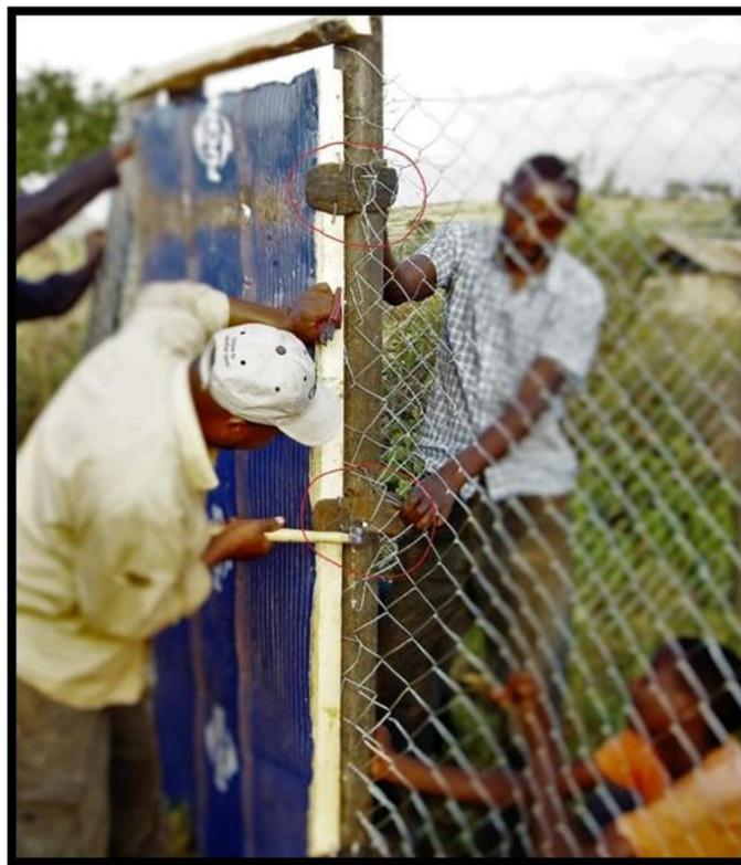
**Plate 1.** PPB door with hinges made from old Maasai sandal.
