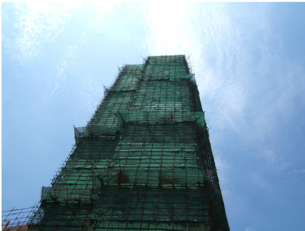
Fig. 25. The use of bamboo as a building//construction material – scaffolding.
