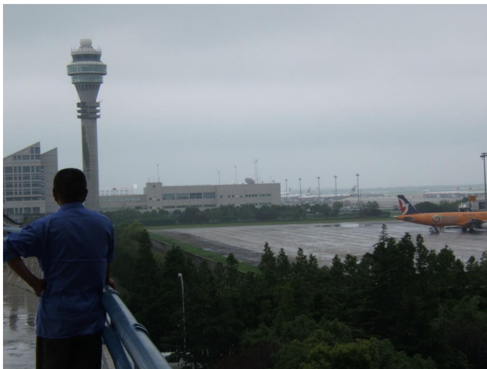
Fig. 10. Airport in Shanghai, China.
