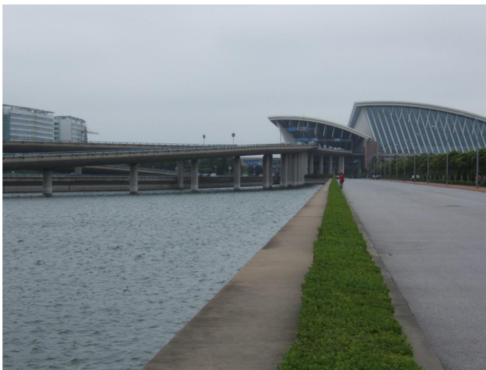
Fig. 6. Airport in Shanghai, China.
