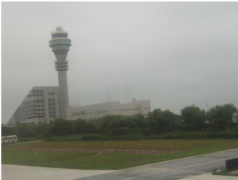
Fig. 5. Airport in Shanghai, China.
