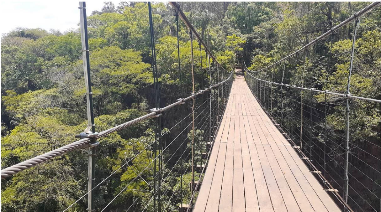
Photo 9. Suspension bridge crossing the valley between the waterfalls.
