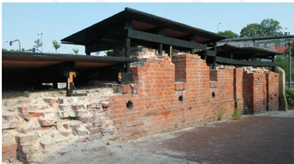
III. 2. Cracow, Rondo Mogilskie, relics of the bastion V "Lubicz". Provisional protections of the crumbling and devastated crowns of the walls (photo by J. Czechowicz)
