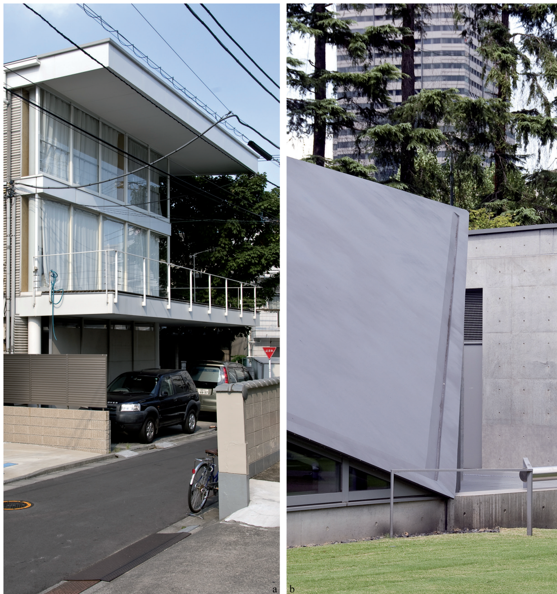
III. 3a) Curtain Wall House, Shigeru Ban, 1994–1995 (photo by author, 2012); b) DesignSight 21_21, Tadao Ando, 2007 (photo by author, 2012)
