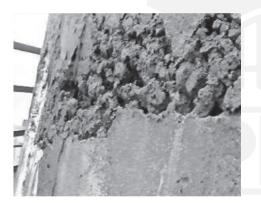
Ill. 13. Insufficiently compressed concrete at the joint of tier of concreting
