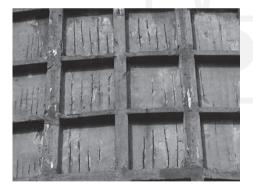
Ill. 11. Steel reinforcement corrosion and destruction of concrete of upper belt of firmness of the cooling tower #4 at Darnytsia Combined heat and Power Plant, protective layer of concrete is lower than designed
