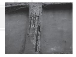
III. 12. Steel reinforcement corrosion and destruction of concrete of vertical ribs of prefabricated slabs of cover of cooling tower #4 at Darnytsia Combined heat and Power Plant, protective layer of concrete is lower than designed
