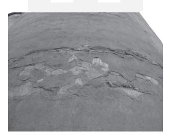
Ill. 16. Scaling of protective layer of concrete with stripping and corrosion of steel reinforcement on the surface of silage walls
