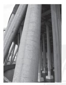
Ill. 7. The lengthwise and cross-cut cracks in pillars of leaning colonnade of cooling tower station #5 of Rivne Power Station
