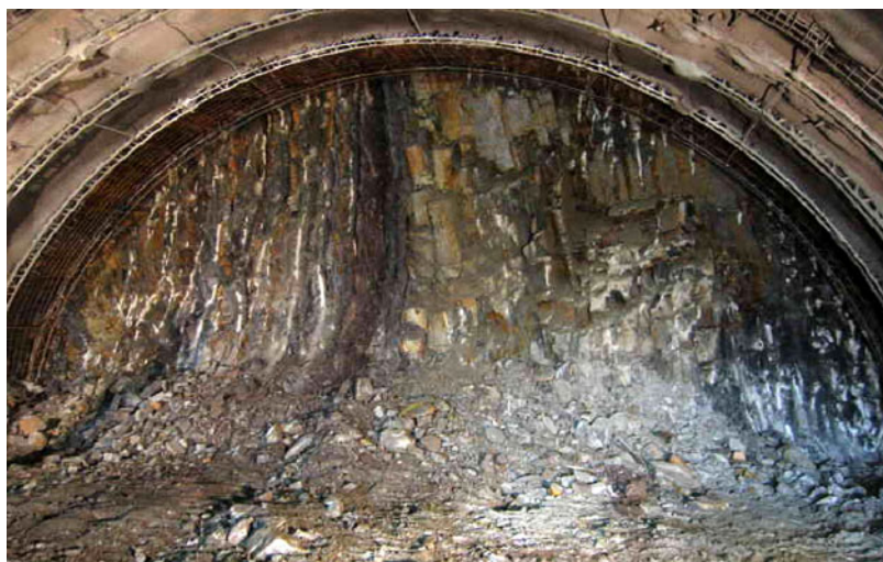
Fig. 2. Tunnel face with typical distribution of strata
