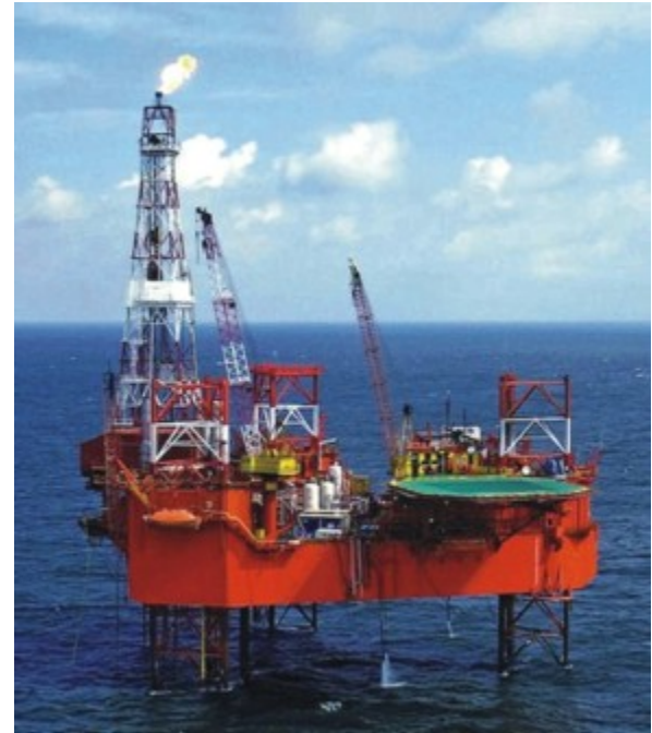
Fig. 5. Drilling platform on Baltic sea.
