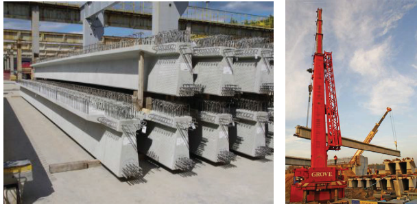
Fig. 2. The storage and assembly of a T-shaped beam [www.sibet.com.pl, www.pw-comfort.com.pl]
