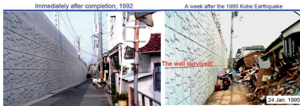
Fig. 6. Geosynthetic reinforced structure (GRS) before and after the Kobe earthquake (Tatsuoka, 2008).
