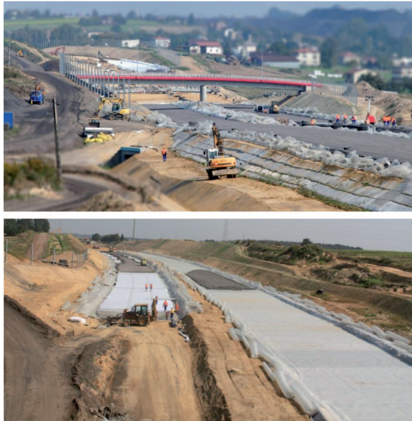
Fig. 2. Highway base reinforcement at Motorway A1 near Gorzyczki, Poland.
