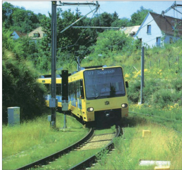
Fig. 1. City railway Stuttgart, Germany. Example of a greened up geogrid reinforced soil structure (1990).
