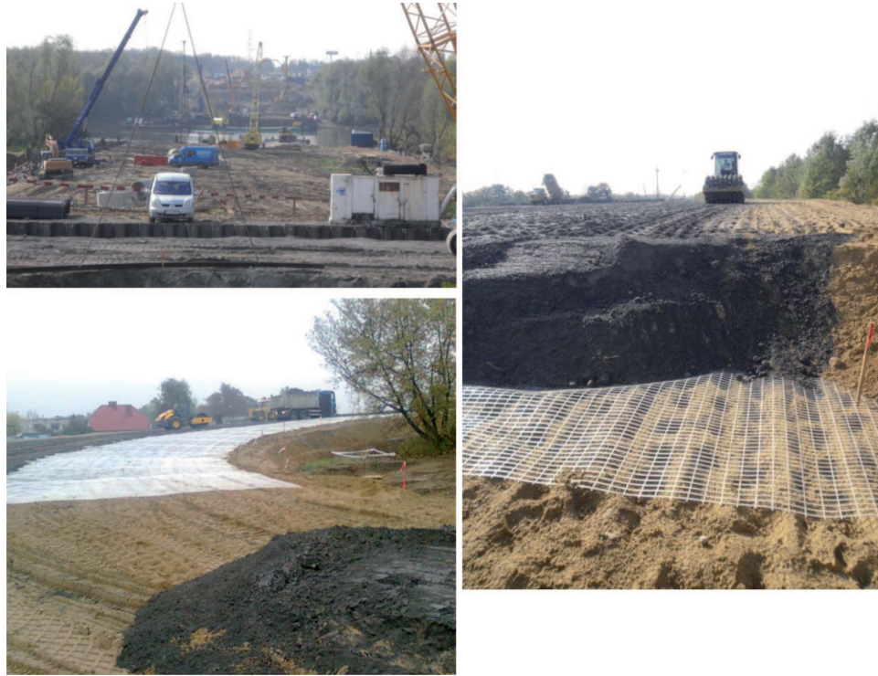
Fig. 3. Embankment reinforcement with geogrids at North Bridge, Warsaw, Poland.
