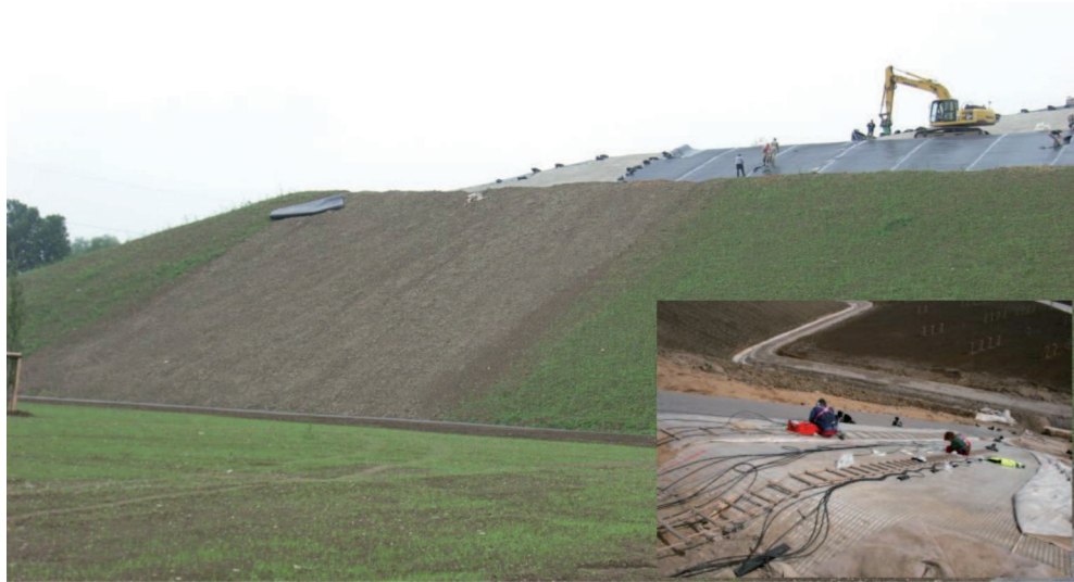
Fig. 15. Creep monitoring of veneer reinforcement at Sudamin landfill, Germany, 2008.
