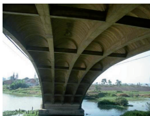
Fig. 2. Elevated view of the superstructure
