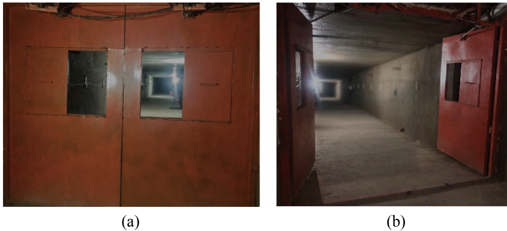
Fig. 4. Field experiment of mine air door
