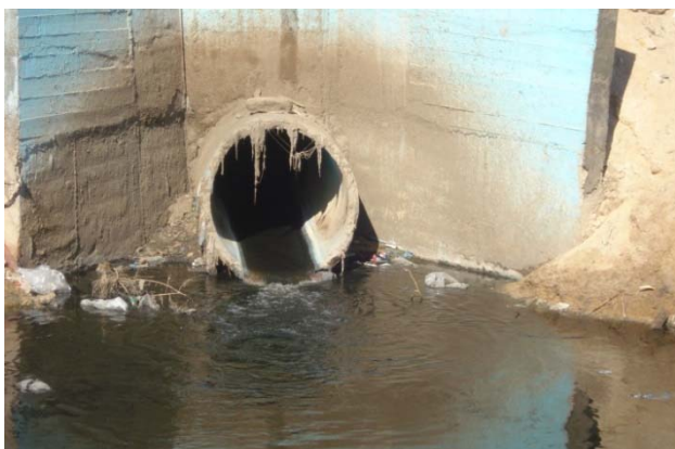
Photo 6. A point of discharge of domestic wastewater in the canal (phot. B. Remini)
