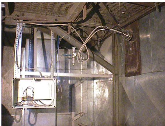
Fig. 6. Fibre probes mounting for: a) wall burner, b) tangential burner
