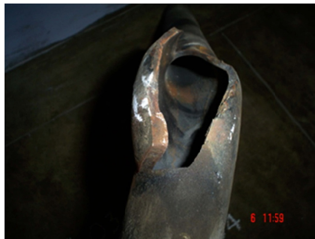
Fig. 1. Failure in inlet pigtail pipe bend
